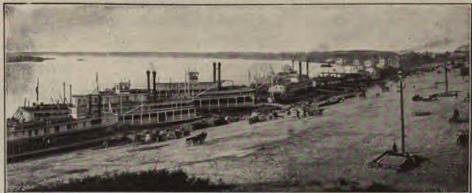
The Mississippi river front at Memphis, Tenn., looking up the river. On the left are small steamboats. In the center is a wharf-boat which takes the place of a wharf, and beyond are larger side-wheeled steamers. It is impossible to build wharves here because of the rising and falling of the river. Merchandise is received on the wharf-boat or piled on the landing, as you can see in the picture. As the Mississippi rises the boats land higher and higher up the bank, until finally they reach the telegraph poles.
